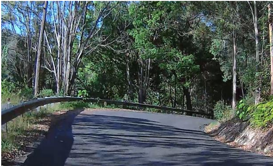
Photo 7: Example of inadequate delineation of curves (no CAMs)
