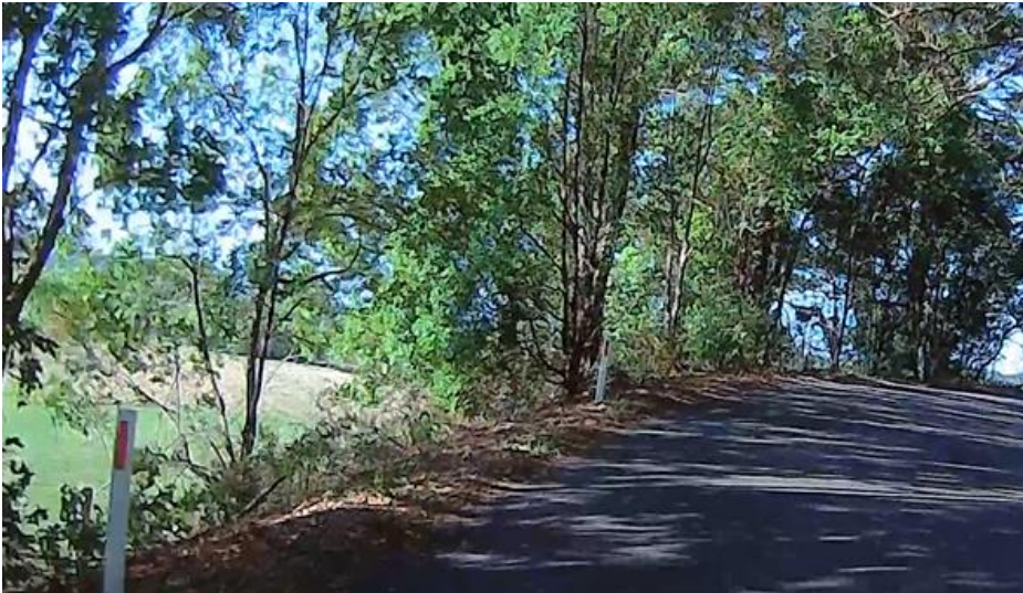
Photo 8: Example of roadside hazards – steep bank down from shoulder
