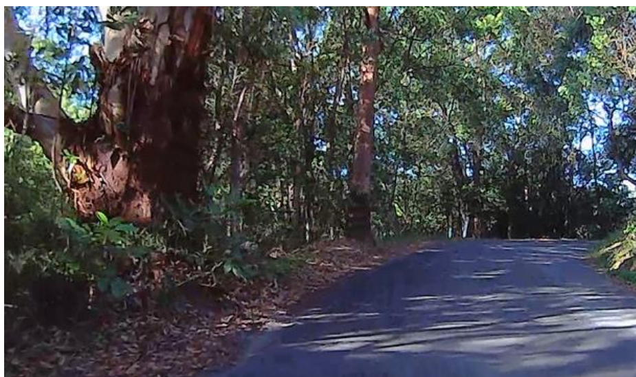
Photo 9: Example of roadside hazards – large trees near road edge
