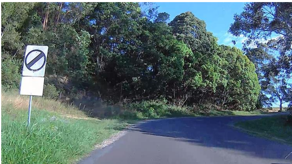
Photo 17: Superseded speed zoning sign; 'Drive to Conditions' sign is totally illegible
