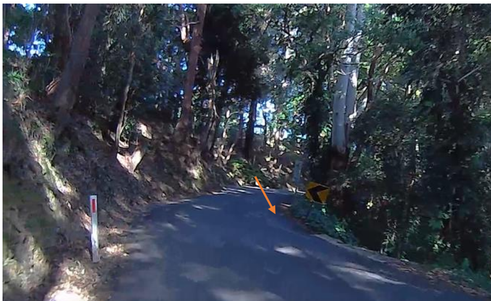
Photo 18: The "slip" at Ch. 1250 – one lane; faded edge line; incorrect use of CAMs
