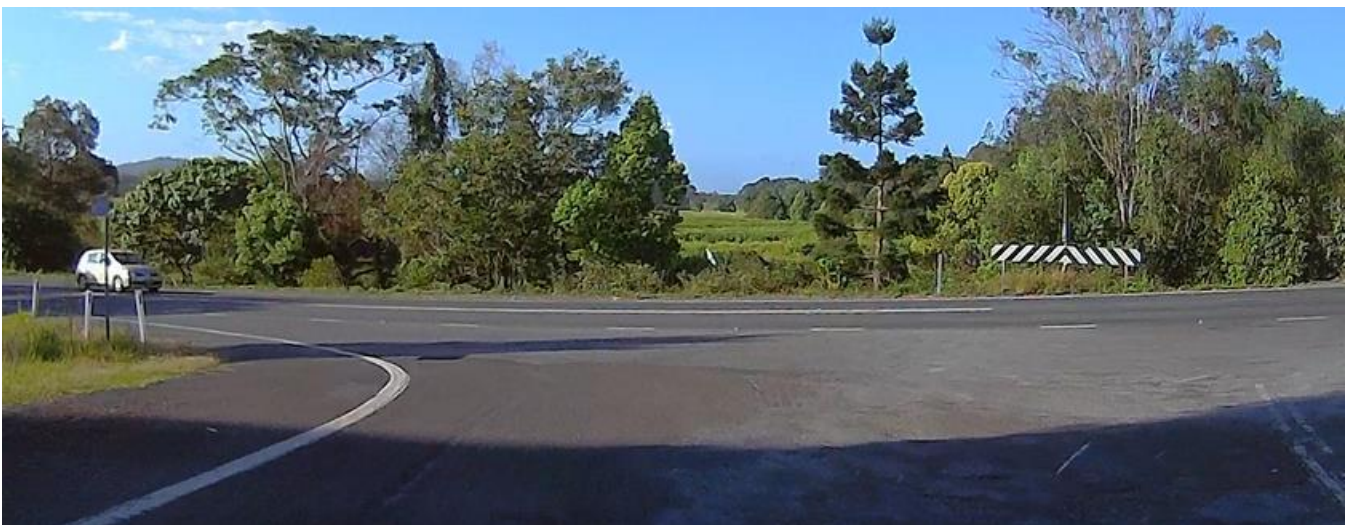
Photo 15: Example of lack of intersection signs/lines – Mullumbimby Road (no stop/give way sign, or hold line)
