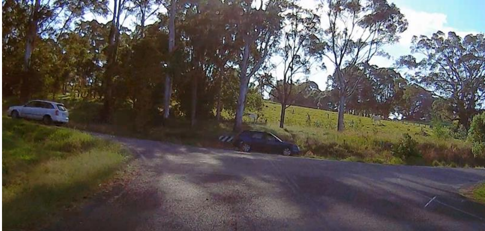
Photo 16: Condition of line marking at Myocum Road intersection (note: no stop/give way sign, or hold line)
