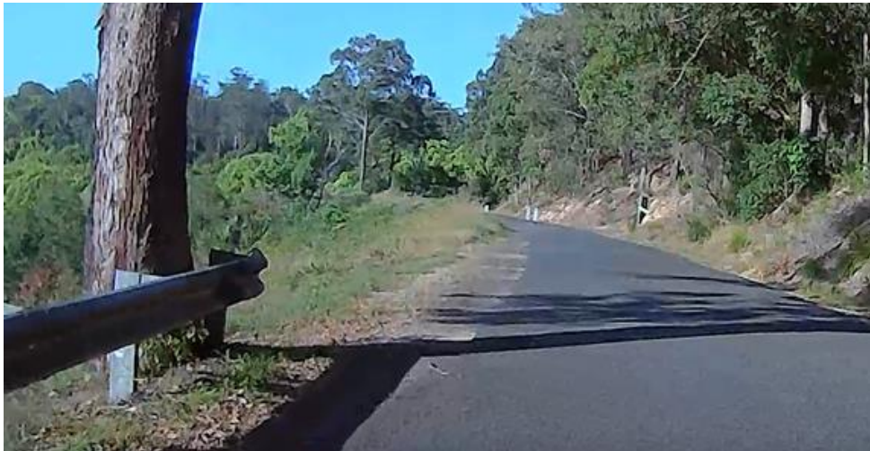
Photo 10: Safety barrier end at tree
